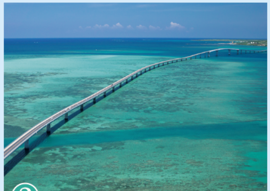
2 The Irabu Bridge
